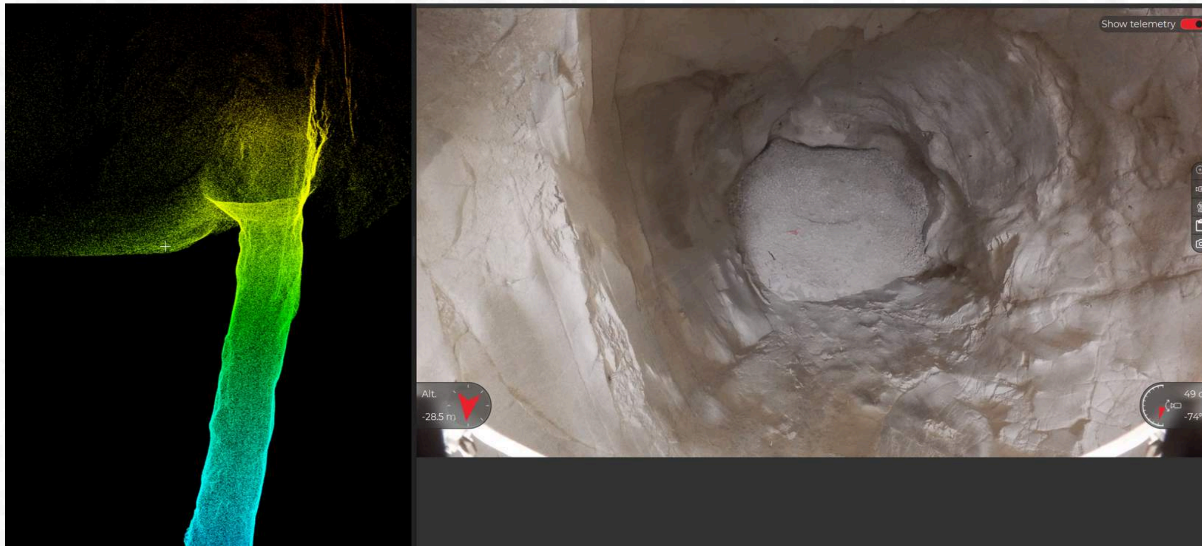
Visual Inspection + Point Cloud
